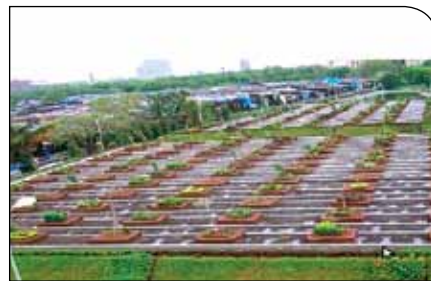
Sewage treatment plant set up at BMC, Mumbai
