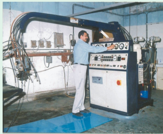
Reaction Injection Mould Facility for Polymerization
