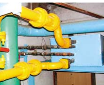
Installation of tube-tube heat exchanger with piping
