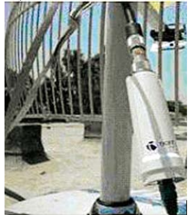
Antenna + ODU – All weather equipment, optimally placed with the antenna
