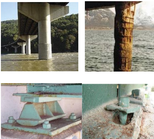
Fig. 1: Realistic deterioration mechanism affecting highway bridge components
