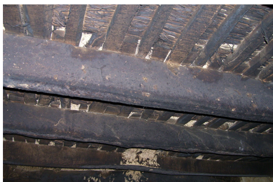
Soot deposition on kitchen walls and kitchen roof due to heavy emissions from the use of cookstoves
