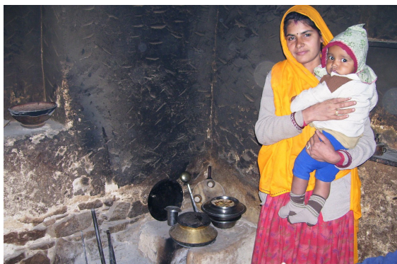
Soot deposition on kitchen walls and kitchen roof due to heavy emissions from the use of cookstoves
