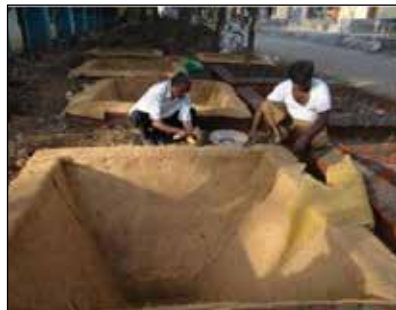
Water storage tanks constructed using natural fibers
