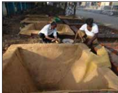
Water storage tanks constructed using natural fibers
