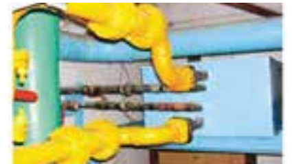
Tube-tube heat exchanger
