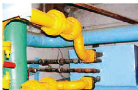
Tube-tube heat exchanger with piping
