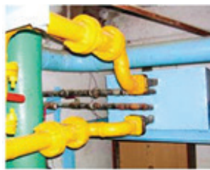
Tube-tube heat exchanger
