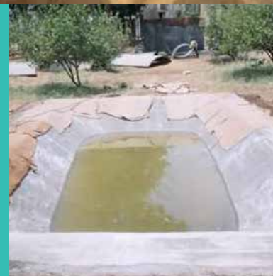
▲ Water storage tanks constructed using natural fibers
