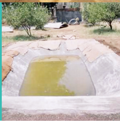
▲ Water storage tanks constructed using natural fibers
