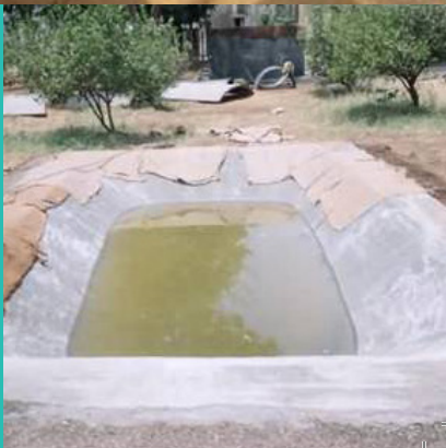
▲ Water storage tanks constructed using natural fibers
